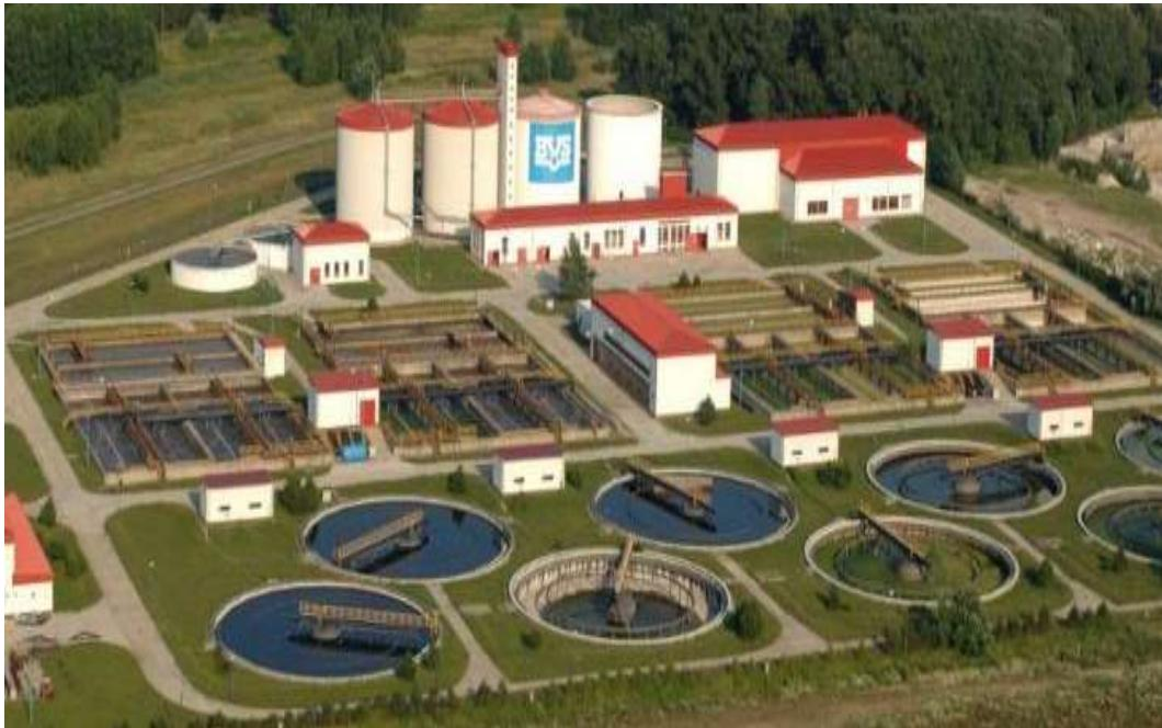
**WWTP** - four parallel lanes (AN1 – AN4), each lane consist of eight sections
